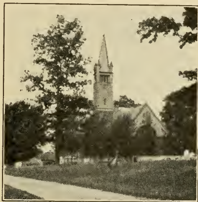
ST. JOHN'S LUTHERAN CHURCH, SINKING VALLEY
